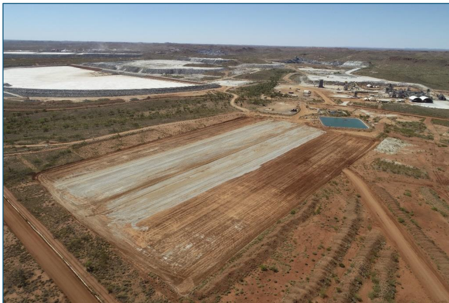
Figure 2 - Early site works have been completed
