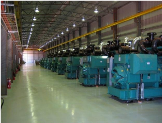
Image: Typical Gas fuelled Engine Shed Layout
