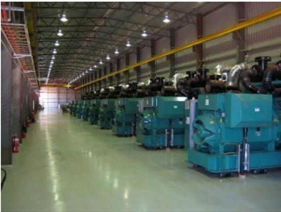
**Image:** Typical Gas fuelled Engine Shed Layout
