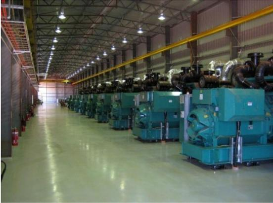
**Image:** Typical LNG-fuelled Engine Layout
